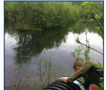
Contractor collects a sample at the effluent of seeps into an Engineered Wetland Remediation System. These seeps emerge from a bluff on the southern boundary of JBER and passively flow into the wetland system. This location is sampled quarterly for chlorinated solvents and petroleum hydrocarbons.
