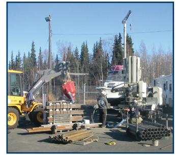
Replacement of monitoring wells at a contaminated site on JBER. Using innovative, green, and sustainable technologies to clean up historical contamination is very challenging in the operational environment. The Team works to minimize impacts to base activities and the risk to human health and the environment.
